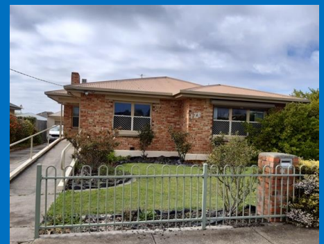
Devonport Shelter - 176 William St.
